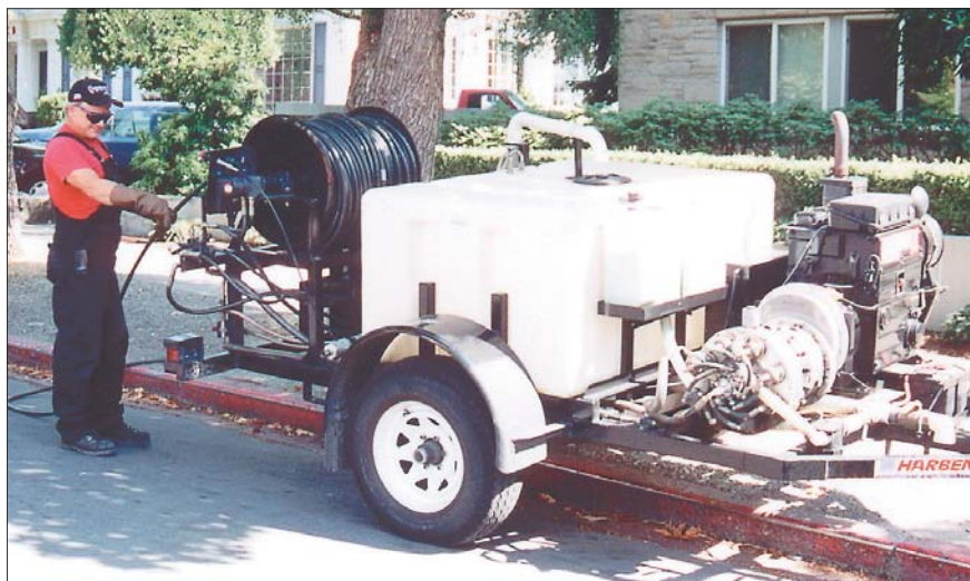
Technician Don Banyai works with a Harben water jetter.
